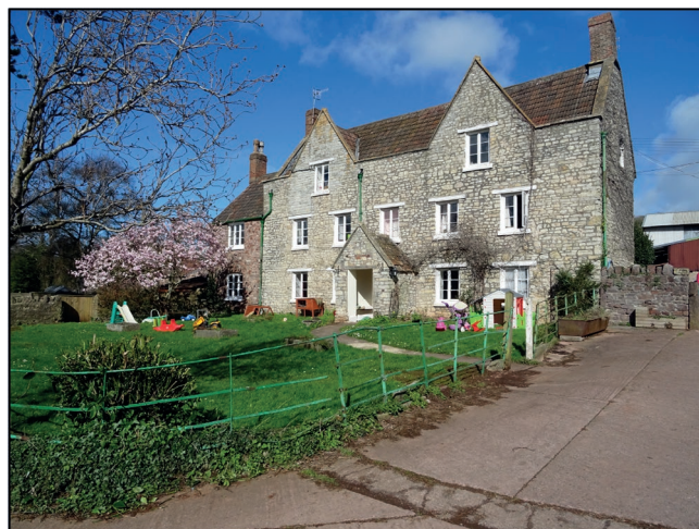
Plate 1 The Grade II Listed Building of Gatcombe Farmhouse.
