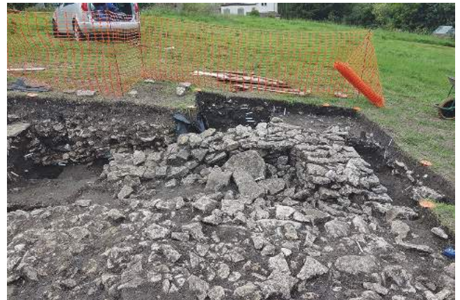
Plate 4 Foundations of Building B's first phase, east face of west gable wall (P.Osborne).
