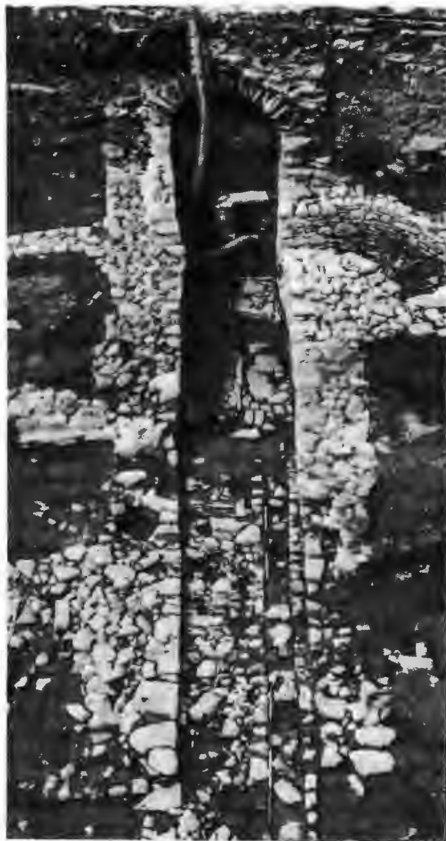
Fig. 8. The Common Slip from the east, showing the arch built across it in the 16th century.
