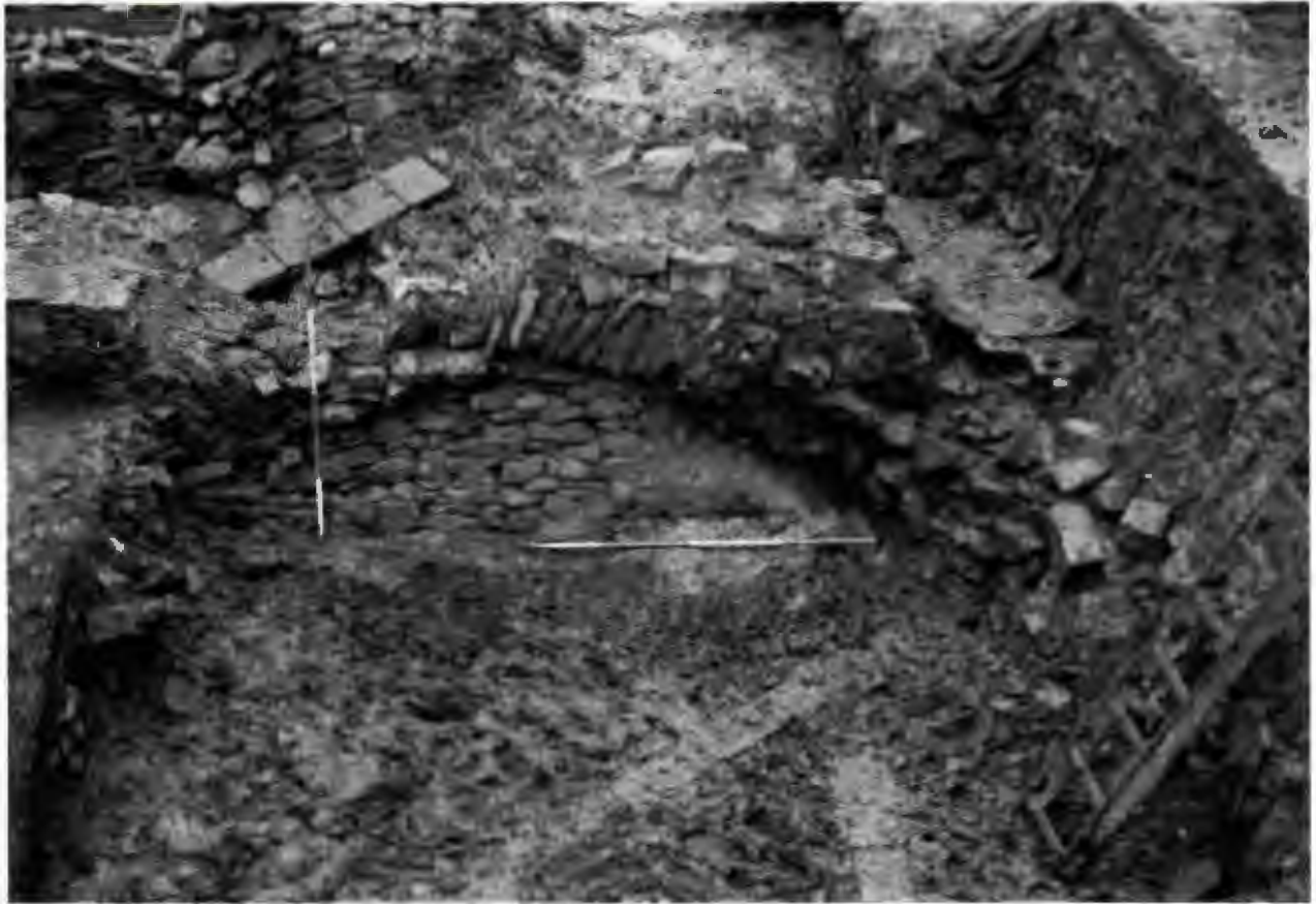
Fig. 10. A construction arch built into the foundations of one of the walls of a quayside building.
