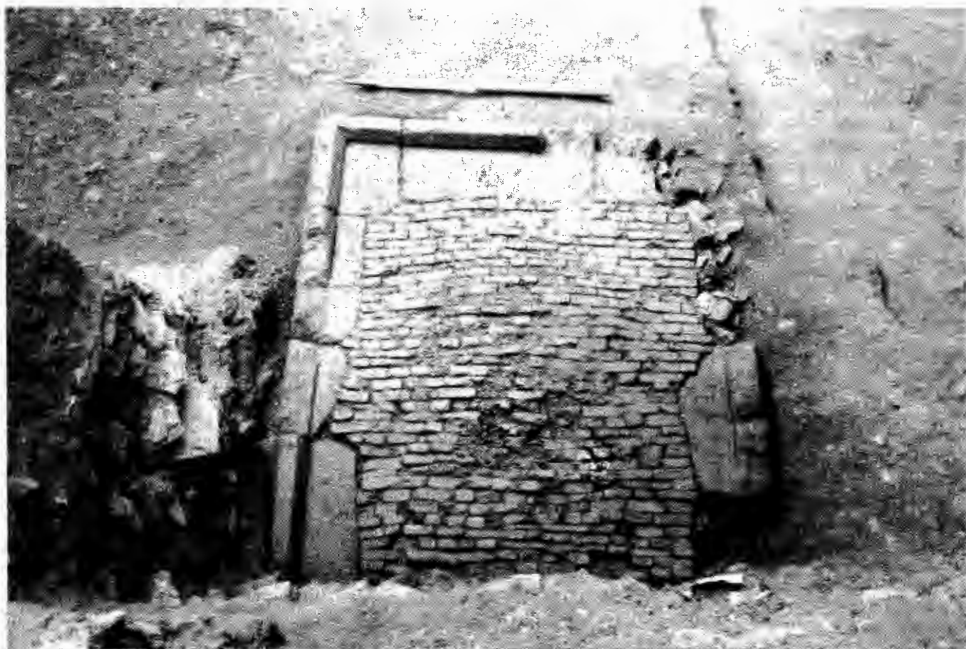
Fig. 3. Upper Maudlin Street, Bristol, 1989: open hearth composed of floor tiles and moulded freestone surround (set in the west end of the hall building). Probably 14th century.
