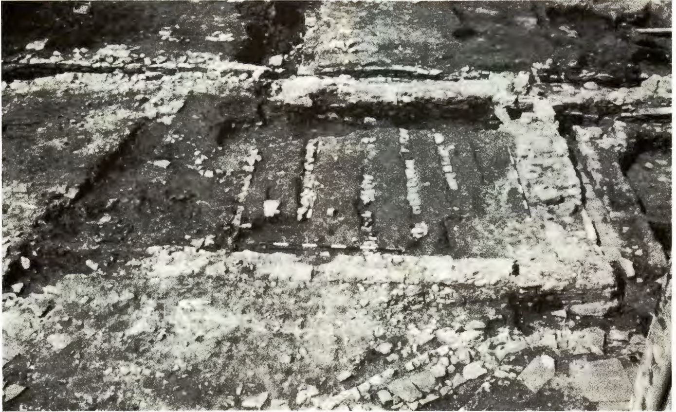
Fig. 18 Vicarage (B3). Phase III — East part of the building showing the foundations of the floor joists. Scales 2m.
