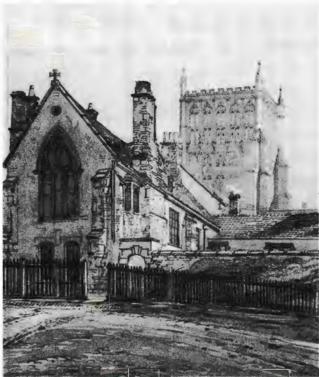
Fig. 2. The Minster House and the cathedral central tower from the south-west by Hugh O'Neill, 1823 (a pencil and watercolour in the Braikenridge collection, M. 1751, Bristol City Museum and Art Gallery).
