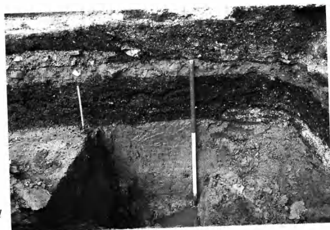
Plate 6 Area 2: west-facing section through the alluvial clay 691 and overlying Period II deposits (scale 1m).
