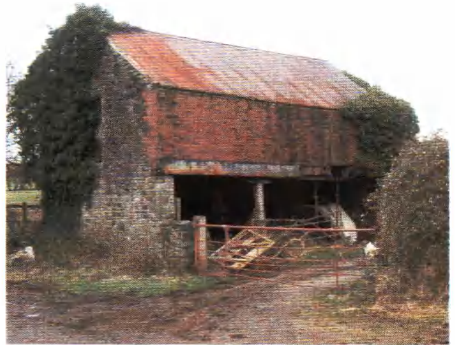
Plate 3 Granary building, looking north-east.
