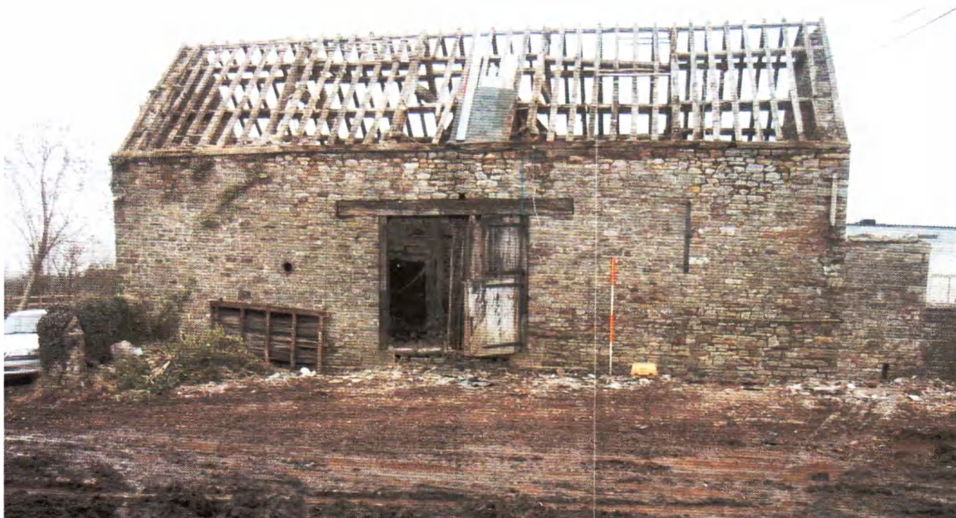
Plate 2 Corn barn, southern side, looking north.
