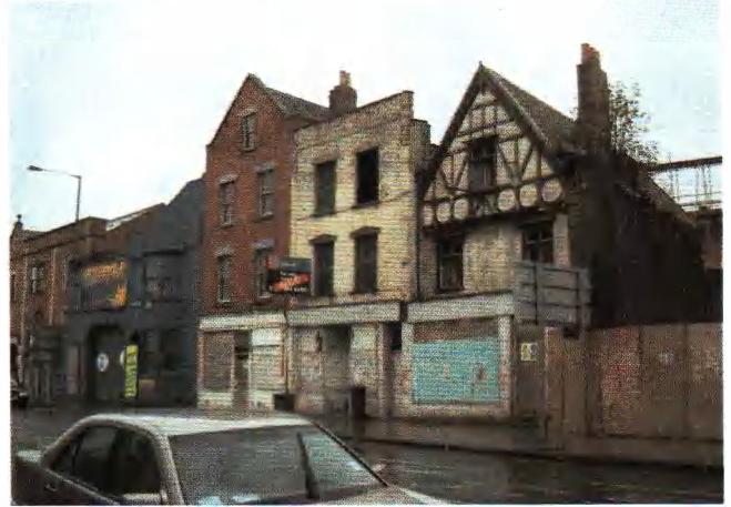
Plate 1 West Street frontage of Nos. 22-30, looking south-east.
