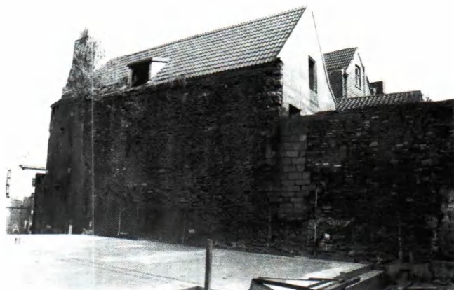
Plate 2 The eastern boundary wall of No. 22 West Street, photographed in April 2003.
