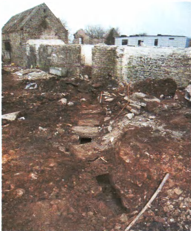
Plate 4 Stone-built drain exposed during groundworks, looking west.
