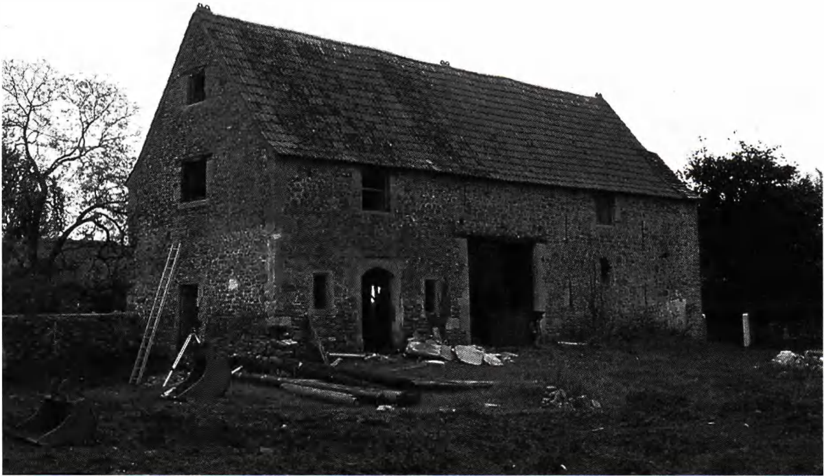
Plate 1 The Barn, looking south-east.
