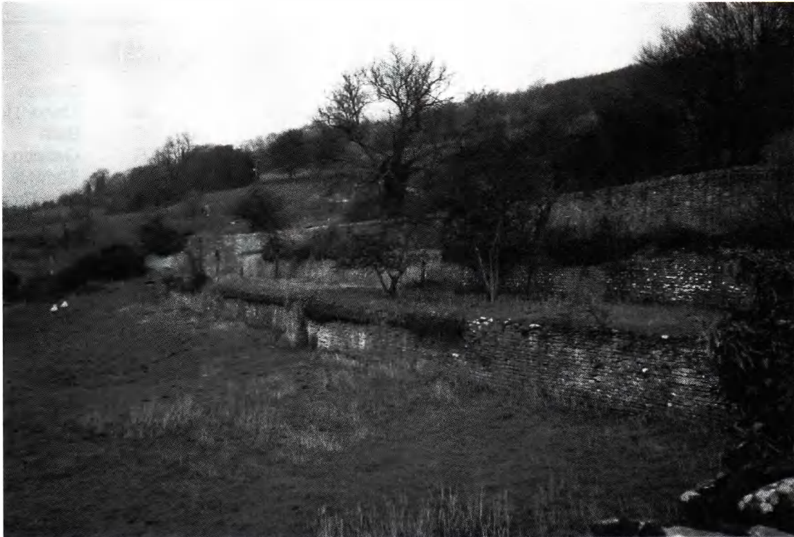
Plate 1 General view of terraces and retaining walls (note doorway opening in middle wall and tufa feature attached to lower wall).
