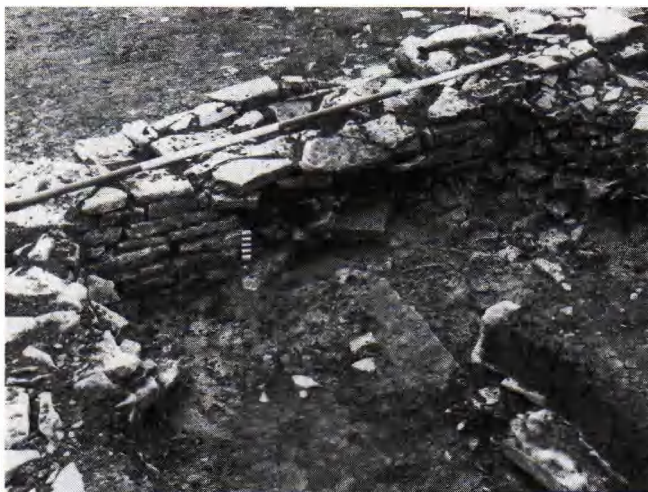
Plate 4 Blocked door in Building C, from the north.
