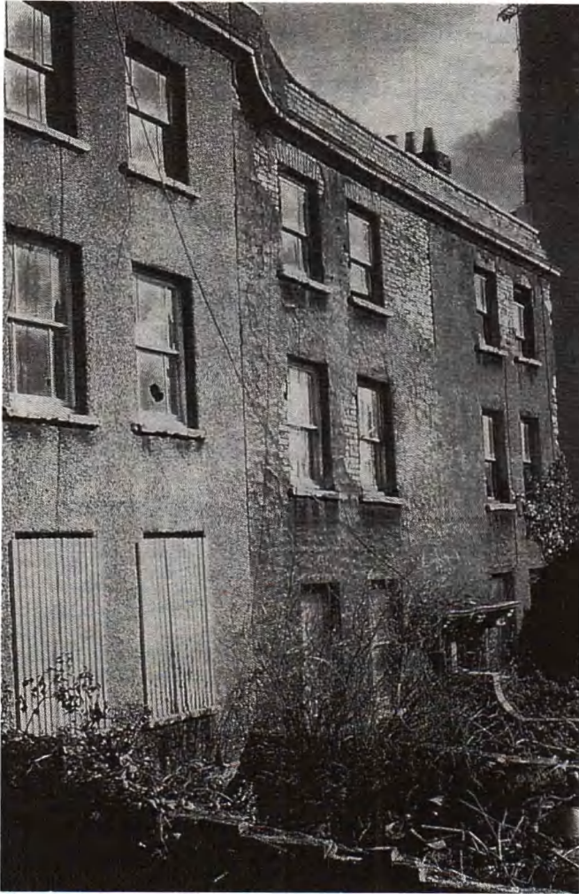
Plate 17 Houses in Pembroke Court, looking south, May 1973.
