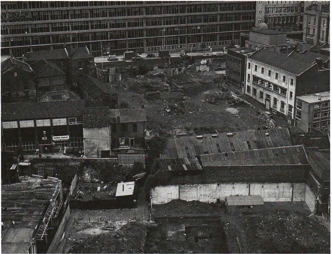
Plate 1 General view looking north showing the 1973 excavations. Part of the 'lower' site around the friary complex can be seen in the bottom of the photograph. Site 1 is in the upper centre of the photograph. The low cliff is defined by the high wall running east/west on the left. The 17th century Abbot's House (unrestored) is the small white building just beyond the wall. The back of the Welsh Baptist Chapel is on the extreme left which, together with the complex of buildings to its right, occupies part of Site 3.
