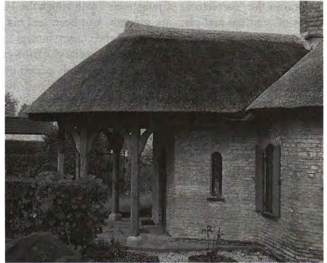
Plate 2 South side of polygonal lodge at 86 Downend Road, probably built for Stephen Cave c.1815. The thatched roof and timber arcade round the porch have been introduced as part of a recent "restoration".
