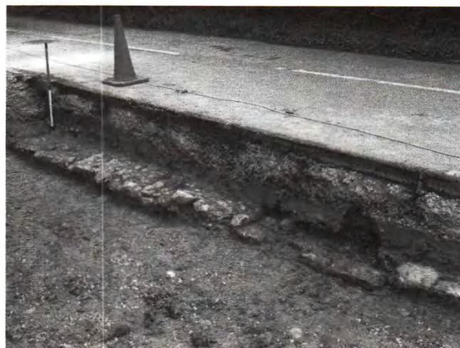
Plate 7 Wall 200, from the south.
