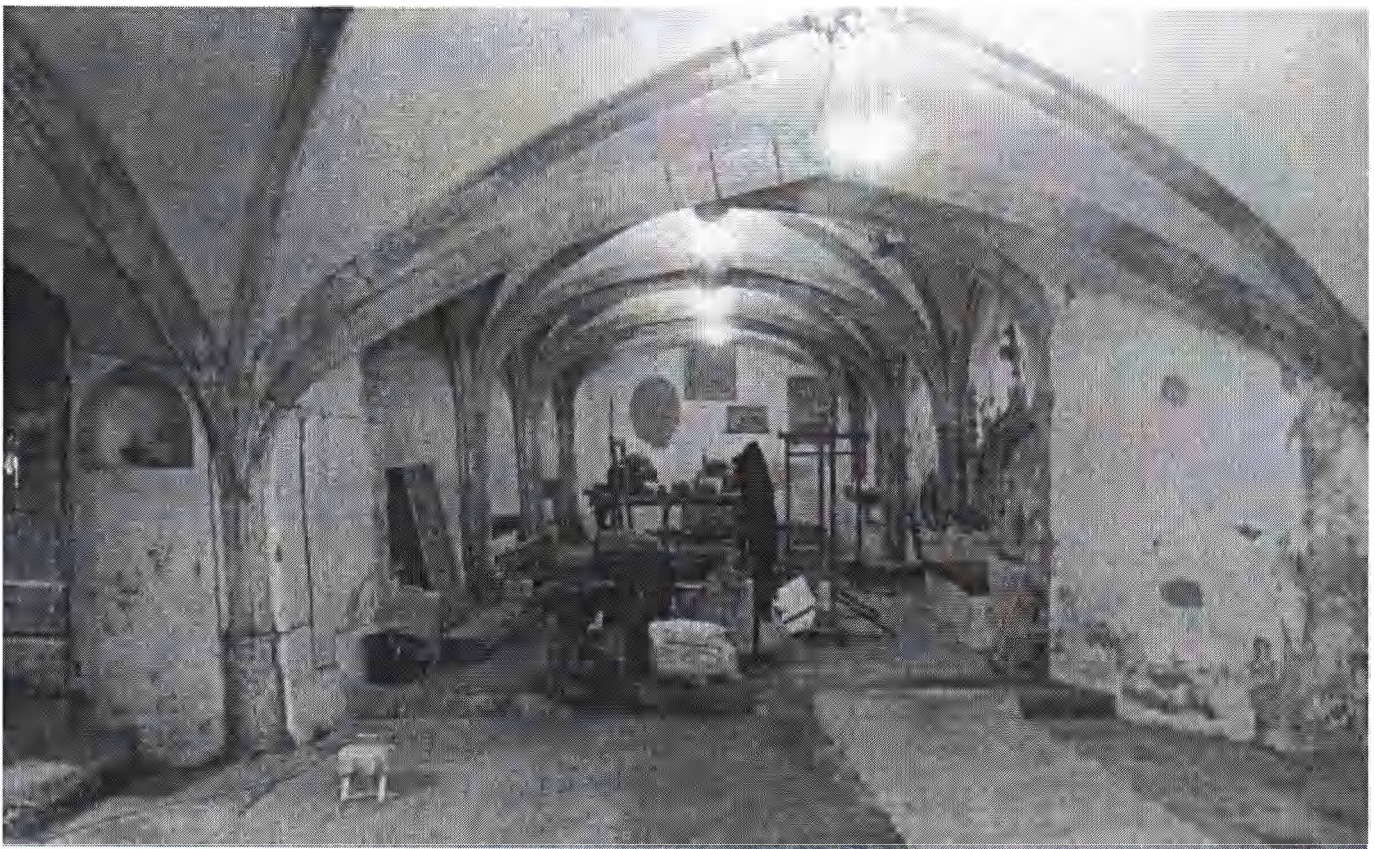
Plate 2 The Crypt before conservation, looking east
