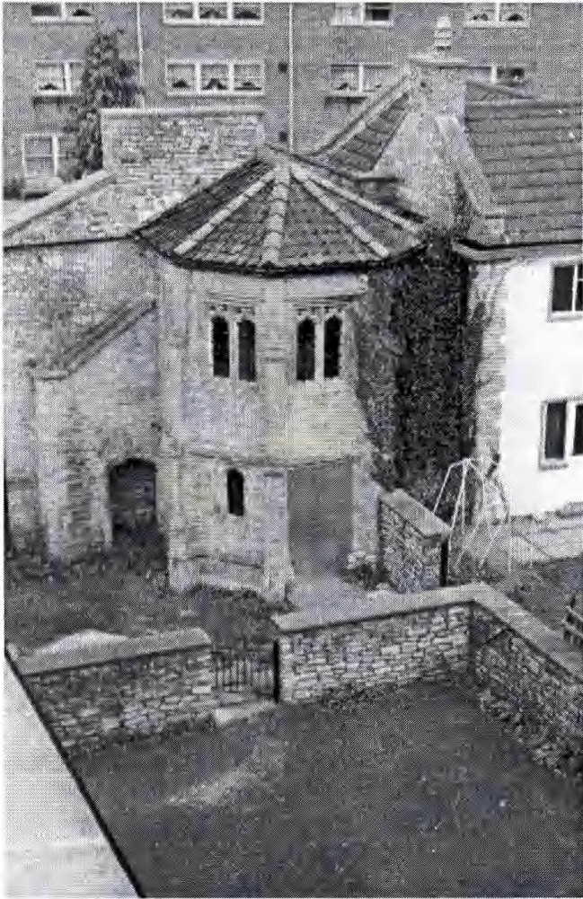
Plate 4 Stair turret on the south wall of the north range of the medieval house, looking north (Period 3B)
