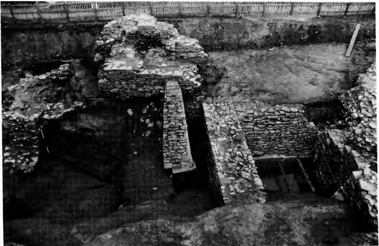
Plate 8 The north wall of the keep, with the revetment, F13 and F13A, on the north slope of the ditch, the 'buttness', F14, and the 'Cross Wall', F12
