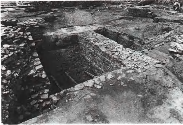
Plate 12 The 'open' area between the 'Cross Wall' F12, and the east wall of the keep, from thenorth-west. The iron bars in the bottom were inserted in 1948 as part of the support for the ditch revetment
