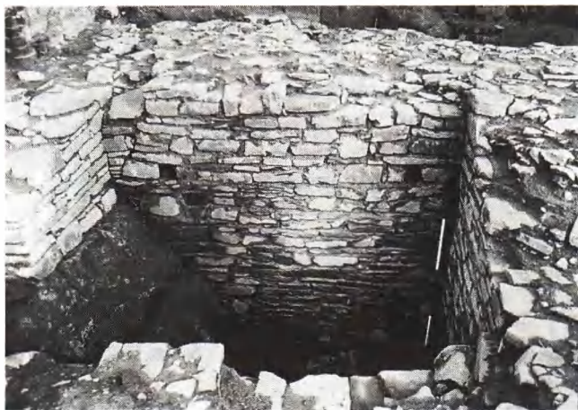
Plate 3 The east side of the shaft, F1, showing the putlog holes
