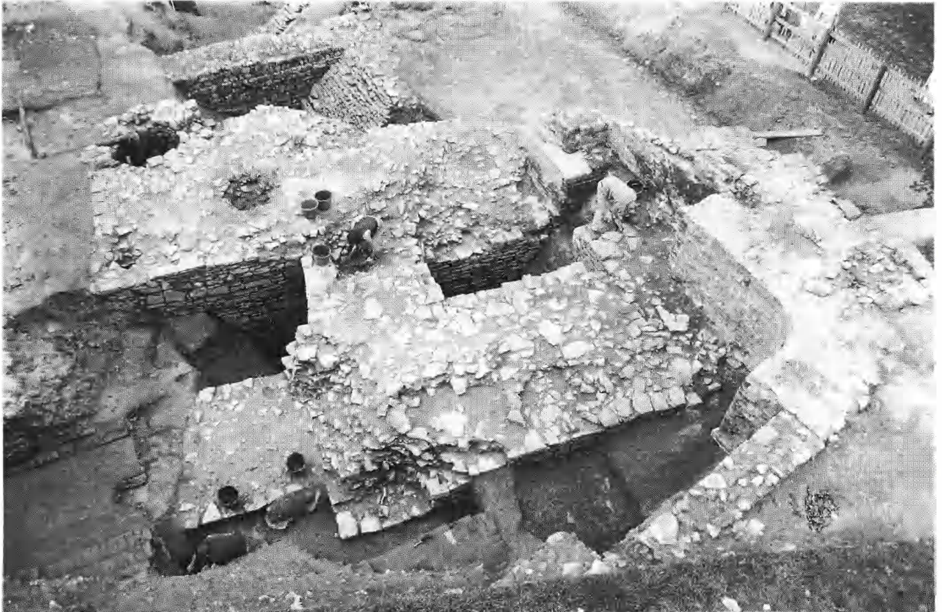
Plate 2 The north-east corner of the keep (Marshall's 'Main Block') from the east
