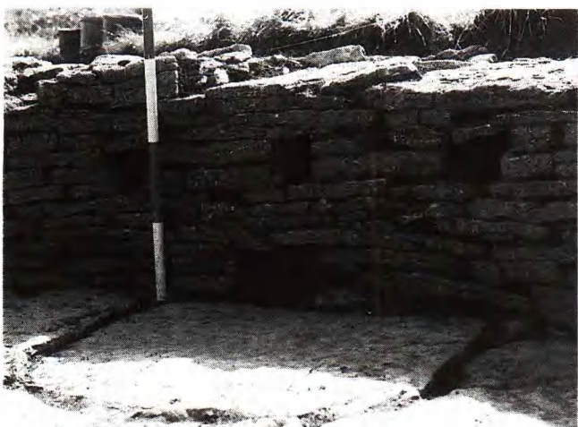
Plate 1b Building 2 - nesting boxes and drain
