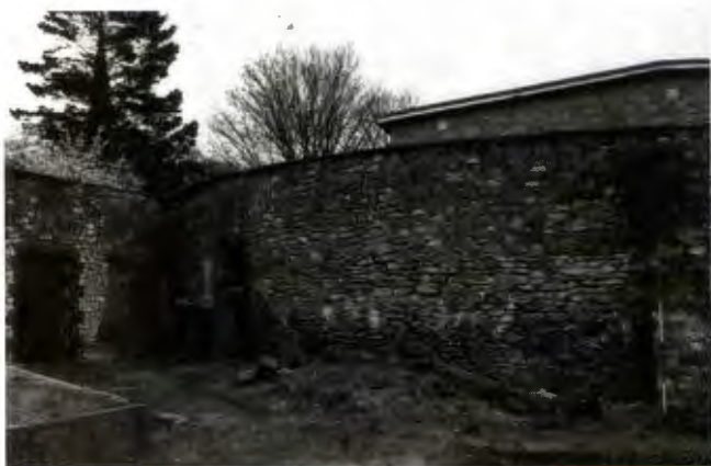
Fig. 3 Stone face of Wall 1
