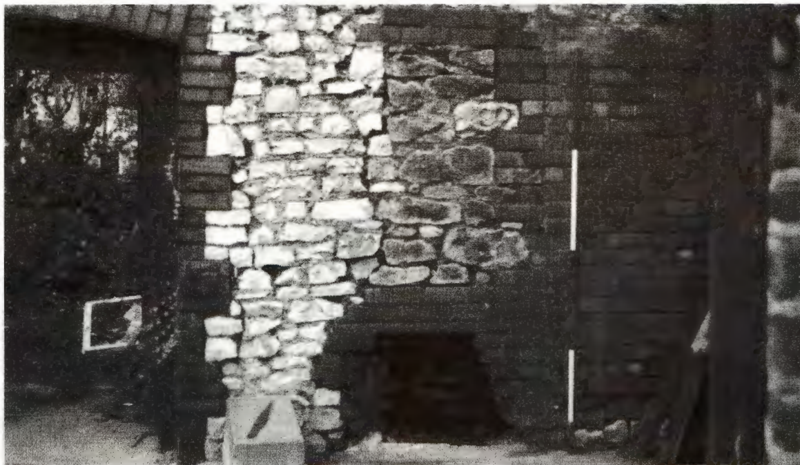
Fig. 5 Blocking and hearth in Wall 2
