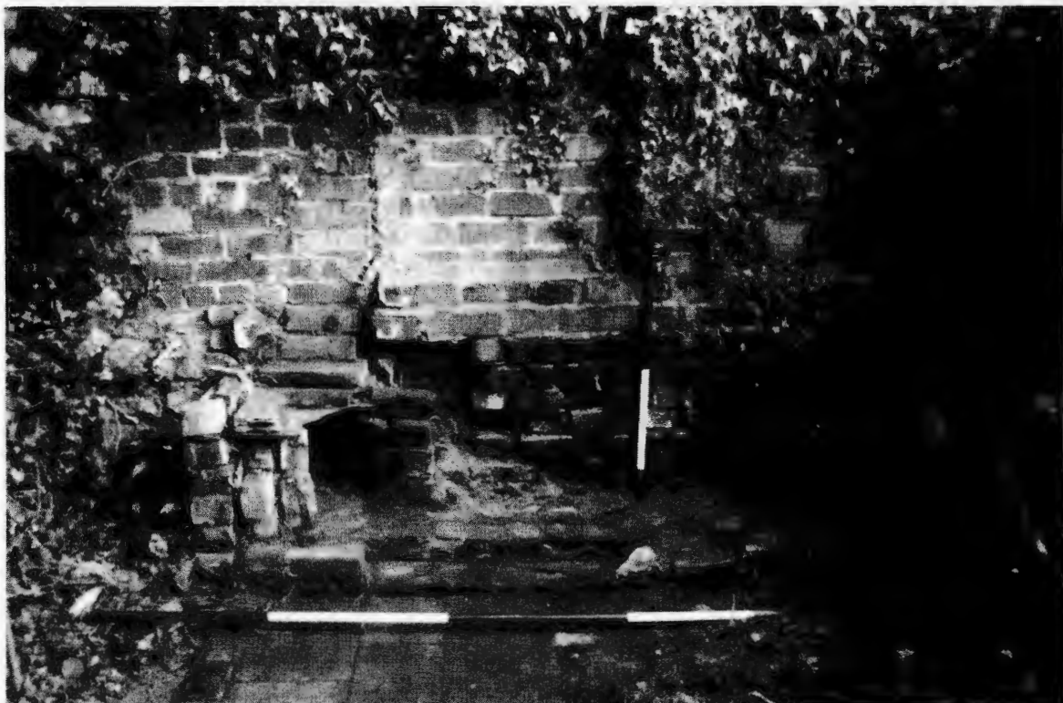
Fig. 9 Flue: Building B1
